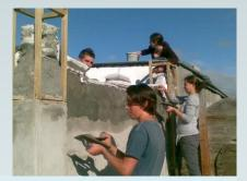
Our regular volunteers picked up from where the Pearson Foundation left off by filling in the many sandbags, extending the walls by laying sandbags in rows and plastering them with cement and concrete mix.
